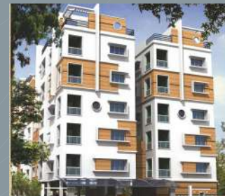
Jains PCH Elite, P.G. Road - Secunderabad
